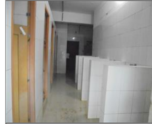
Photo of the sanitary facilities Toilet.JPG
