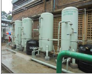
External photo(s) of the production unit(s) Water treatment plant.JPG
